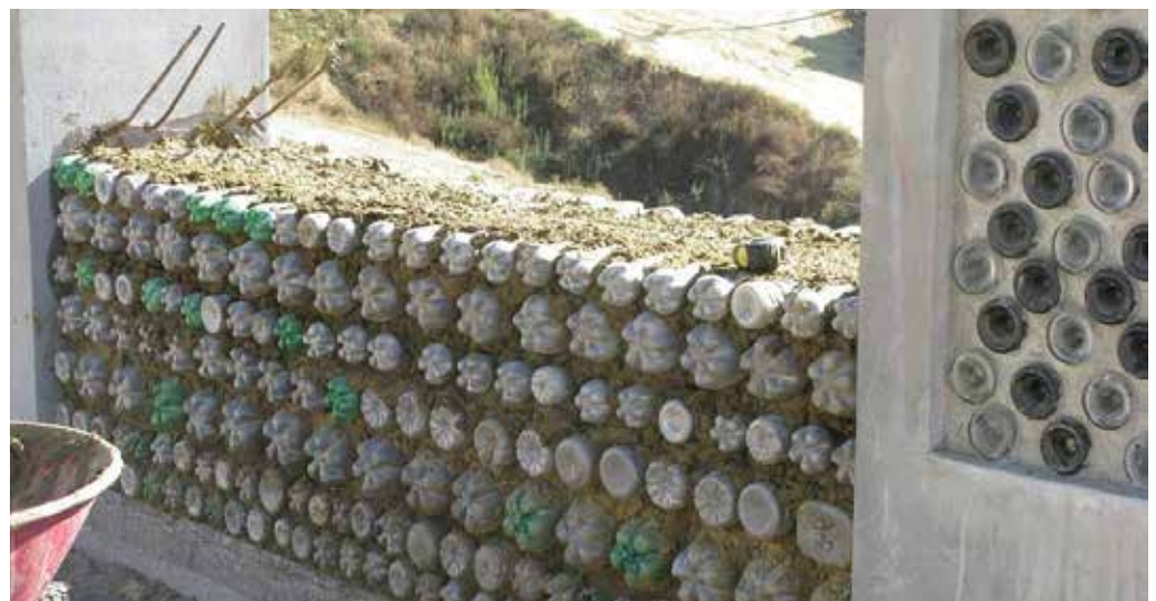
An example of how walls can be built using Ecobricks.
